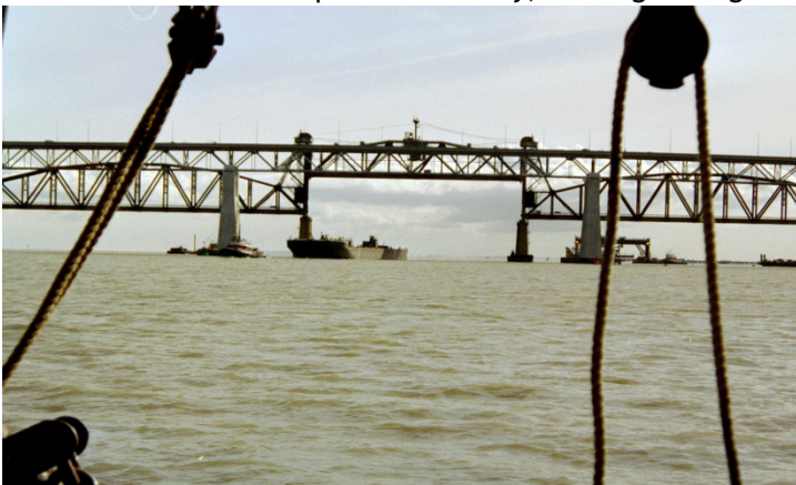
The Benicia Bridge Railroad Bridge
