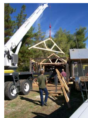
Setting roof trusses
