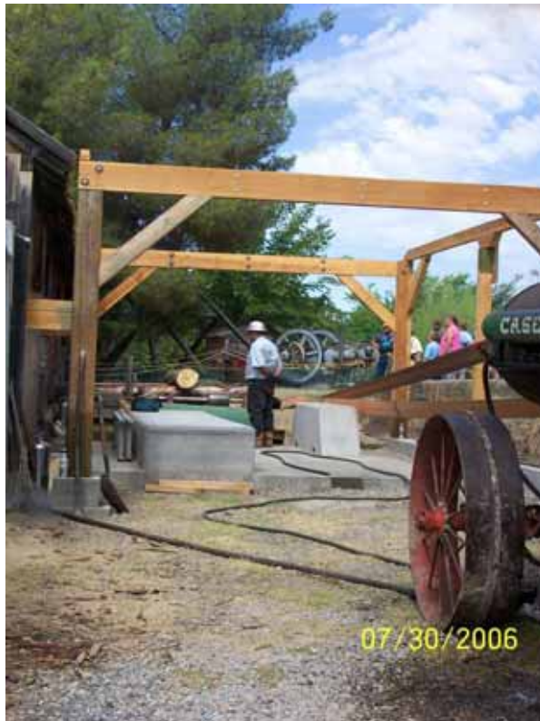
View of future engine room
