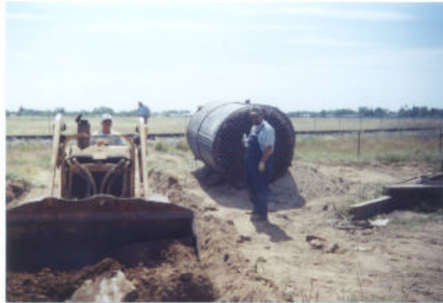
John watching Mike dig the loading trench
