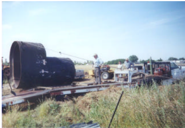
Rolling the boiler onto the equipment trailer
